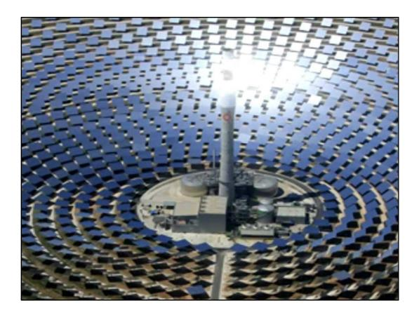
This is another form of Solar power – Concentrated Solar Power, using mirrors and a collector.
