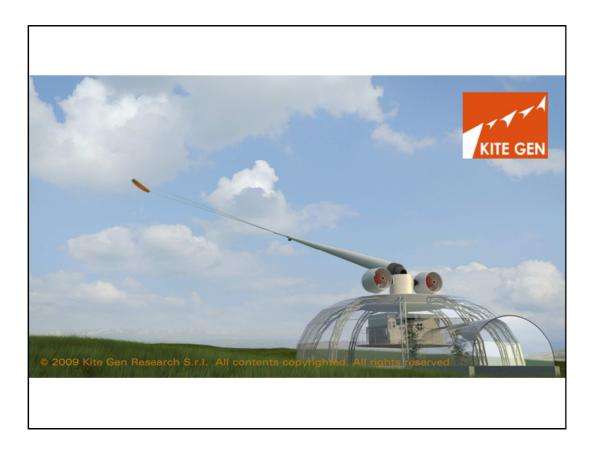
Kite power is another area of development, and Scotland again leads the way in the UK. The principle behind this is to get the kites up into stronger steadier winds, where they can travel at up to 100mph, pulling on the ropes to activate a turbine.
