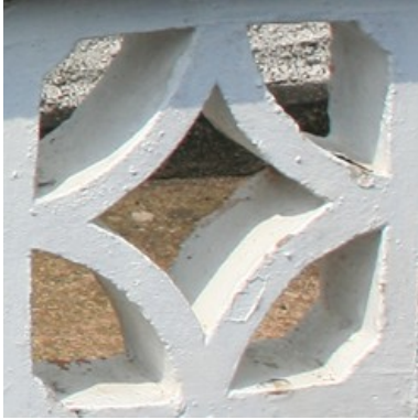
Wall outside 2 Silbury Place
